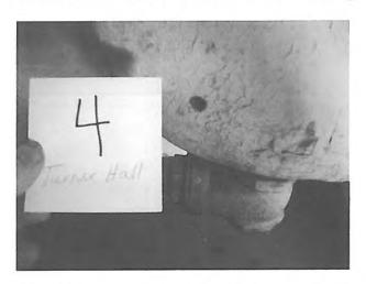
Pipe Fitting Insulation in Mechanical Room which was confirmed to be asbestos containing and is scheduled for removal in June of 09.
